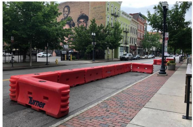
FIGURE 3. Site Plan – Water Barrier Examples (High Volume Roadways):
